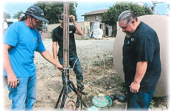
Meter Vendor Testing a Well's Inline Meter for Accuracy
